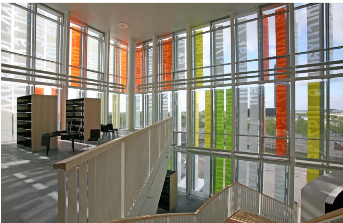
*Ørestadens Gymnasium, Copenhagen, Denmark. - Colt designed and installed 700 laminated and printed bespoke Shadoglass glass louvres over an area of 1700m<sup>2</sup> of façade for shading and ventilation. The different colours, films and frits provide a youthful and playful appearance.*
