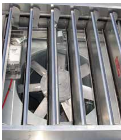
EuroCO as termination piece above a fan (guard removed)
